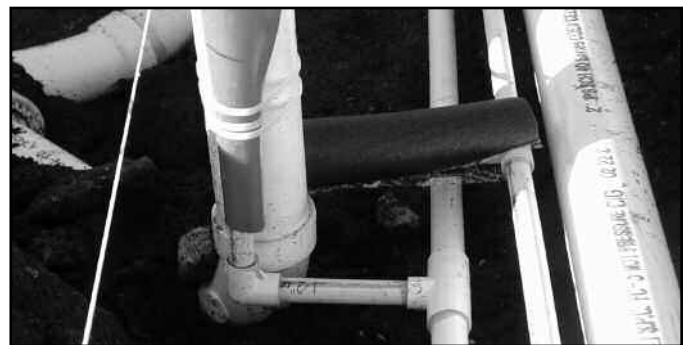
Closeup of FlowGuard Gold joints underslab
