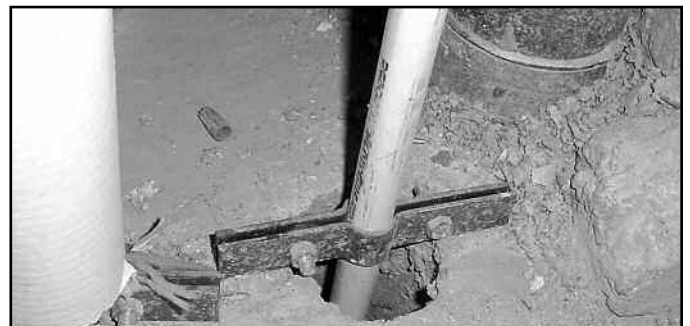
Typical riser supports using FlowGuard Gold pipe.
