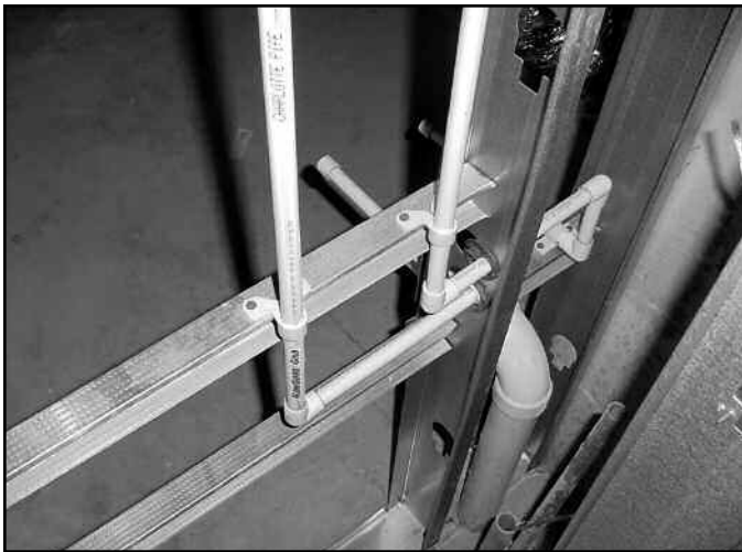
FlowGuard Gold pipe support at metal studs.
